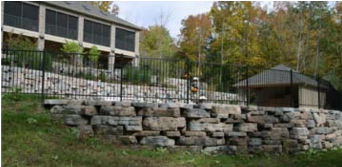
Koudys' goal in the design was to integrate the swimming pool and the cabana structures into a landscape surrounded by existing trees on the steep slope. "We were looking for a wall building material that would allow us to hold back the grade, and would deal with the significant loads that the slope would put on the wall. The goal was to create a structure that was attractive and visually interesting," Koudys said.
